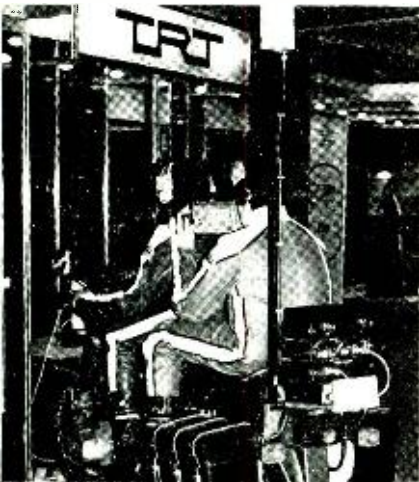
TRT omni-range ENG portable microwave on rear of motorcycle.
